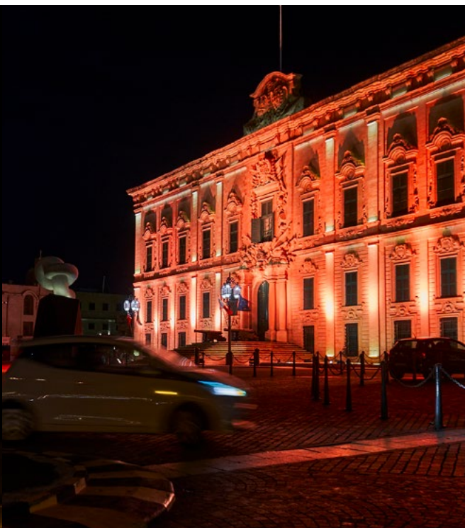
Lighting of public buildings - Castille
